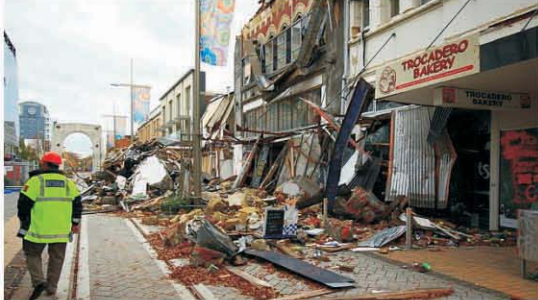
A worker walks along the destruction at Cashel Mall. (Photo by Ross Becker)
